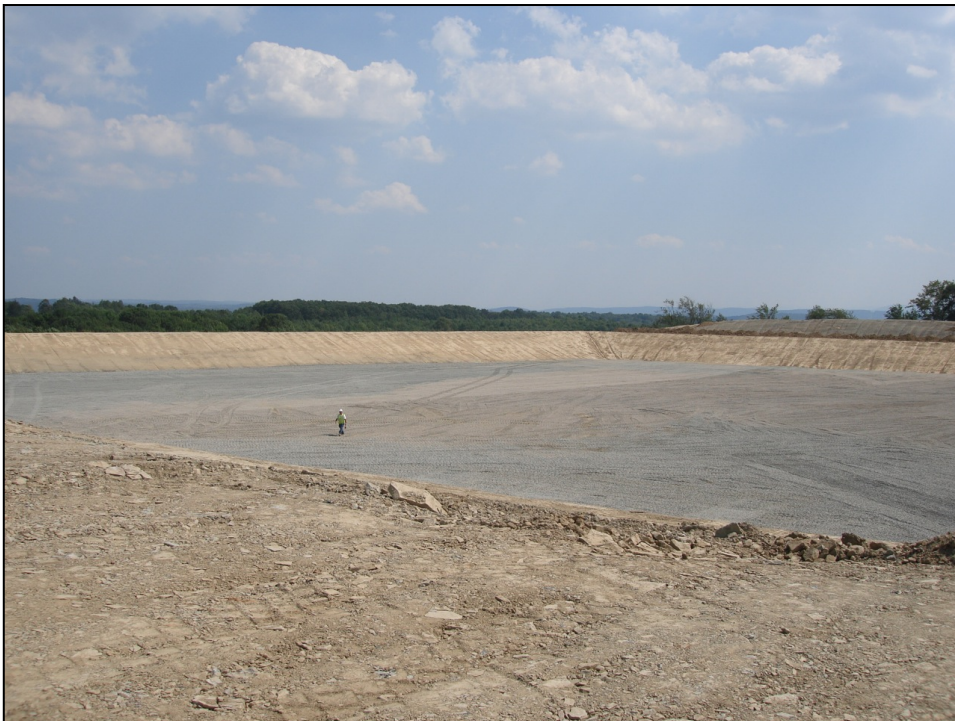
Well Pad Preparation (photo Carol Chock)
